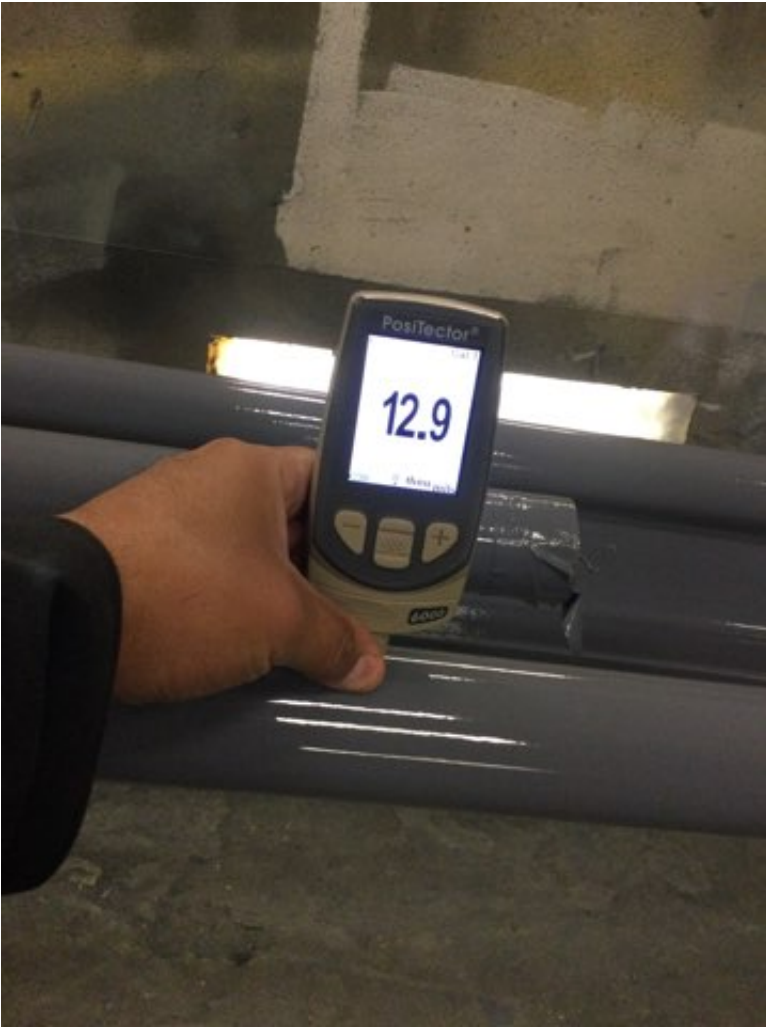
Photo Description: Polyurethane dry film thickness measurement
