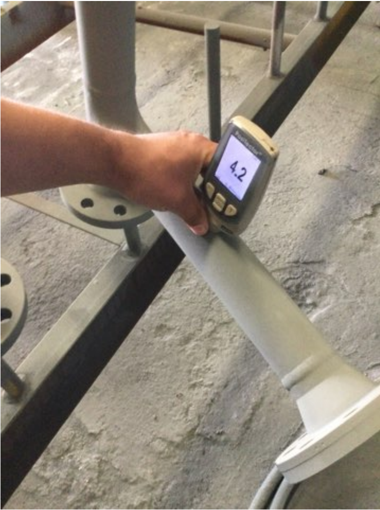
Photo Description: Zinc coating dry film measurement
