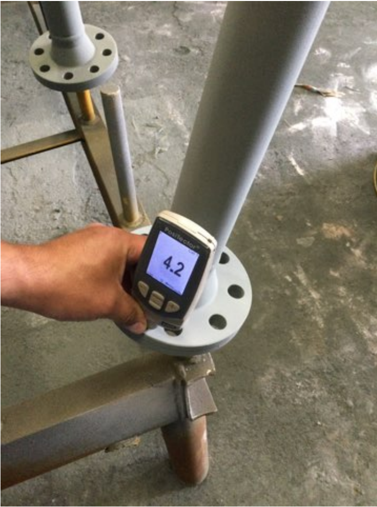
Photo Description: Zinc coating dry film measurement
