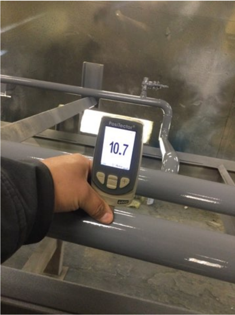
Photo Description: Polyurethane dry film thickness measurement
