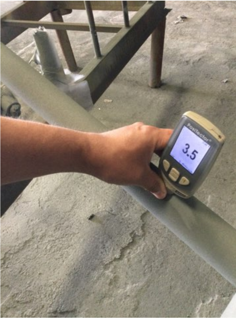
Photo Description: Zinc coating dry film measurement
