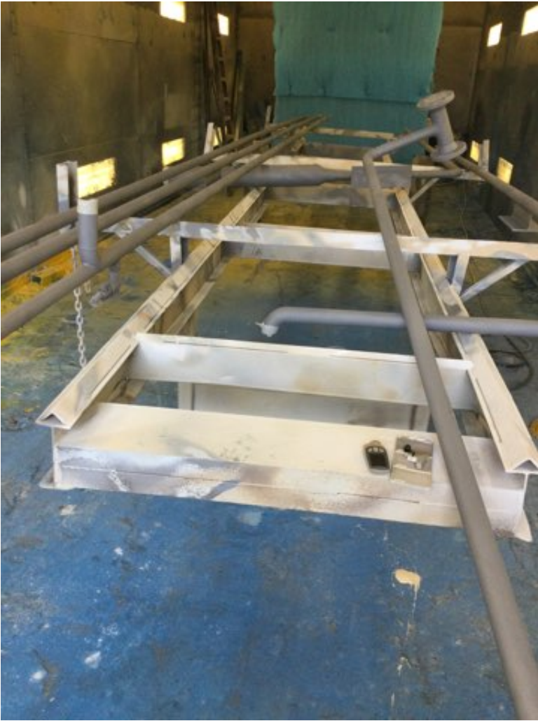
Photo Description: Grit blasted
