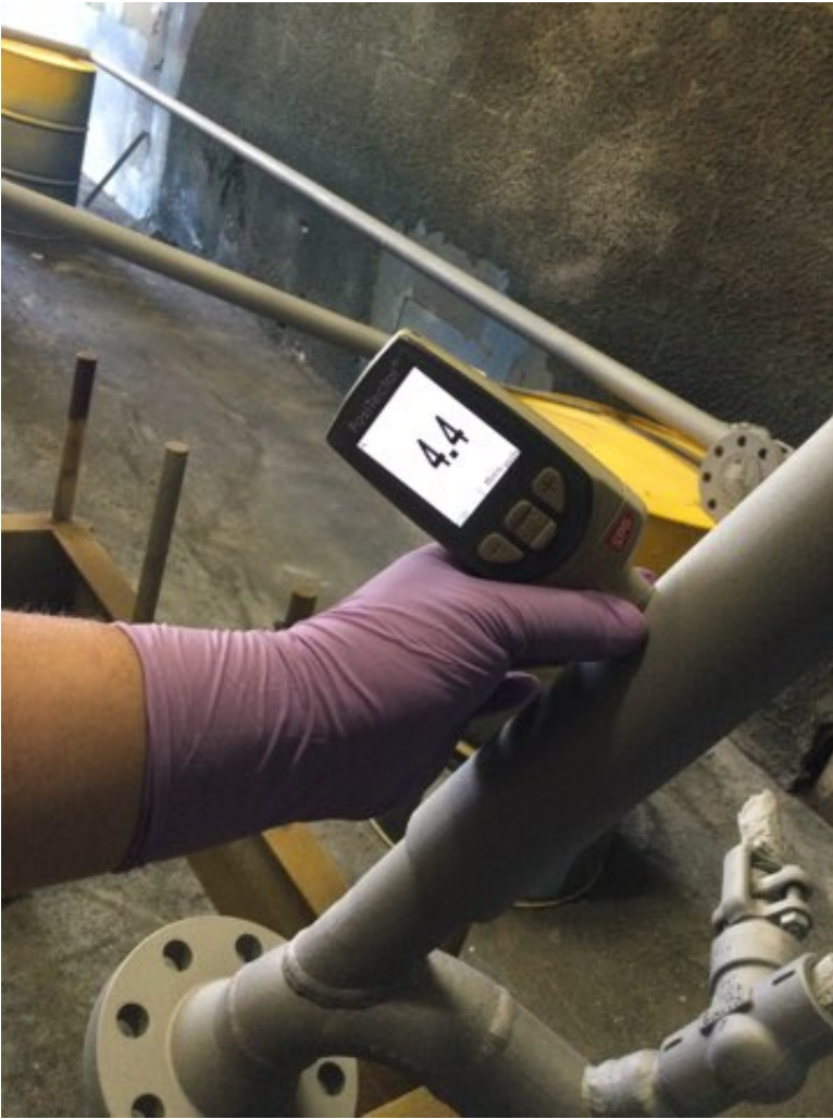
Photo Description: Grit blasted Surface profile measurement
