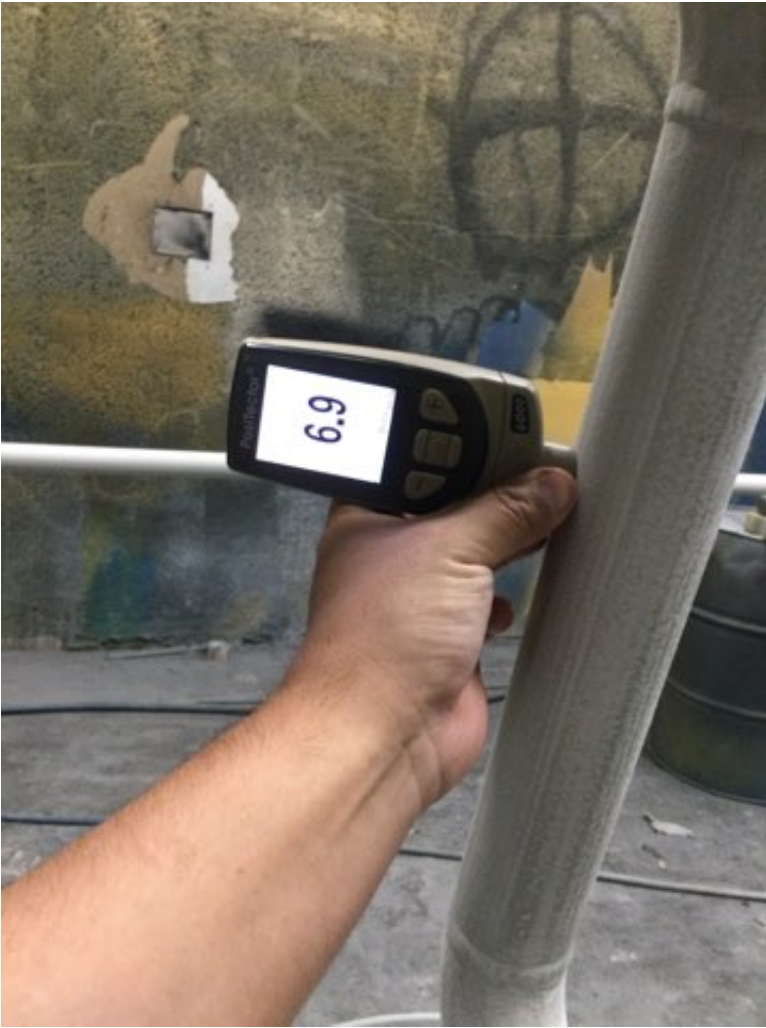
Photo Description: Epoxy dry film thickness measurement
