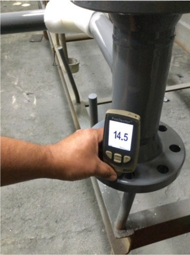
Photo Description: Polyurethane dry film thickness measurement
