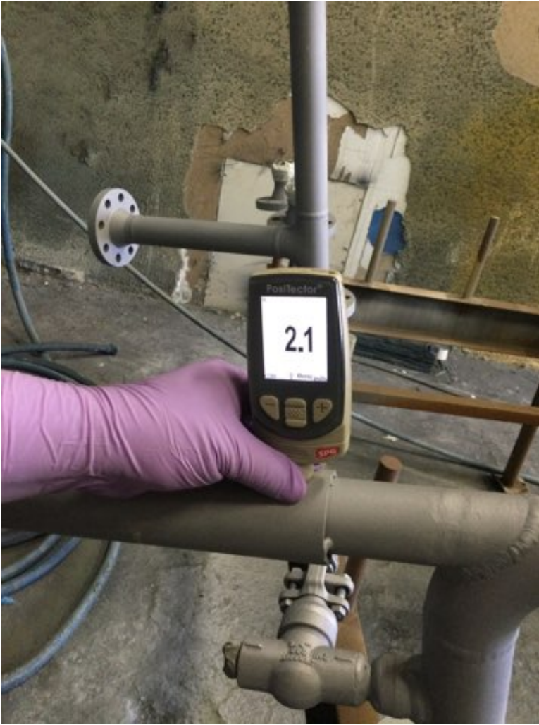
Photo Description: Grit blasted Surface profile measurement
