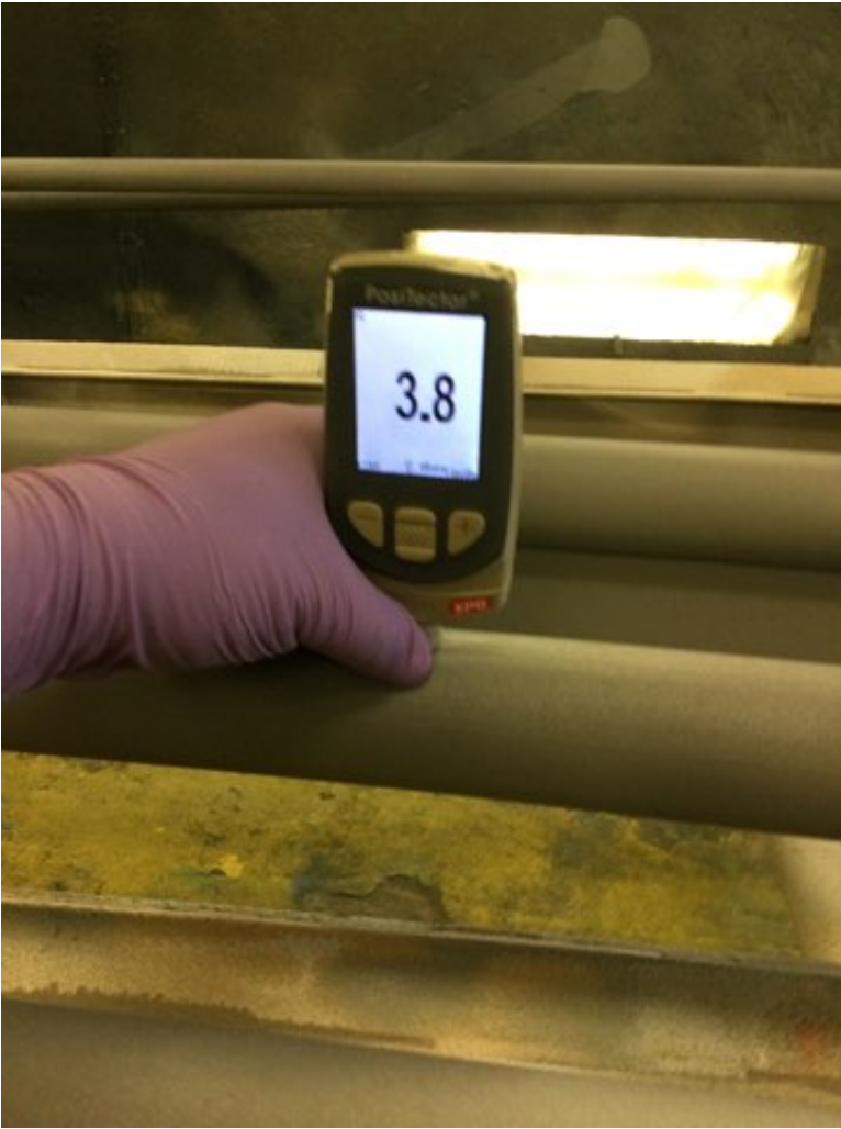
Photo Description: Grit blasted Surface profile measurement
