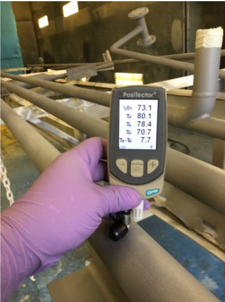
Photo Description: Immediately before zinc primer coating
