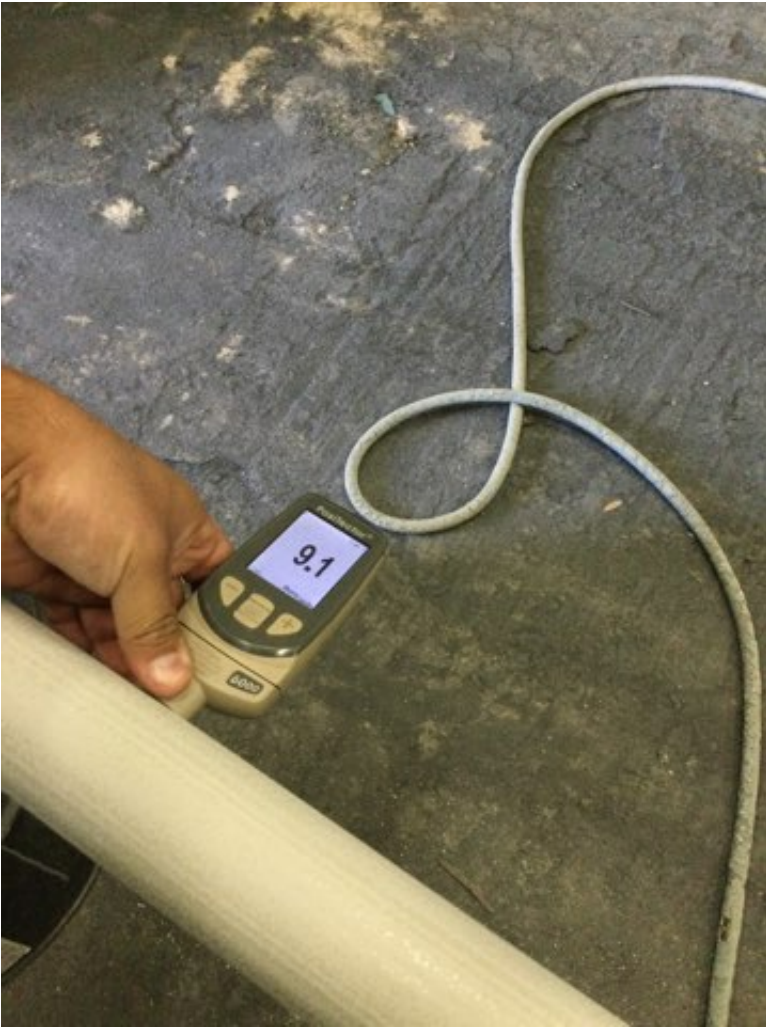
Photo Description: Epoxy dry film thickness measurement
