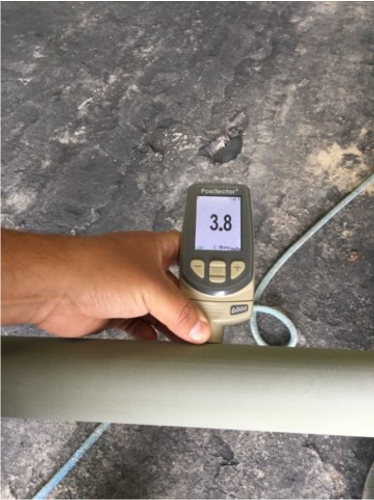
Photo Description: Zinc coating dry film measurement
