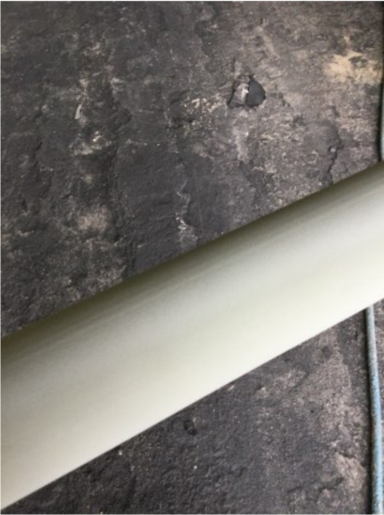
Photo Description: Zinc coating dry film measurement
