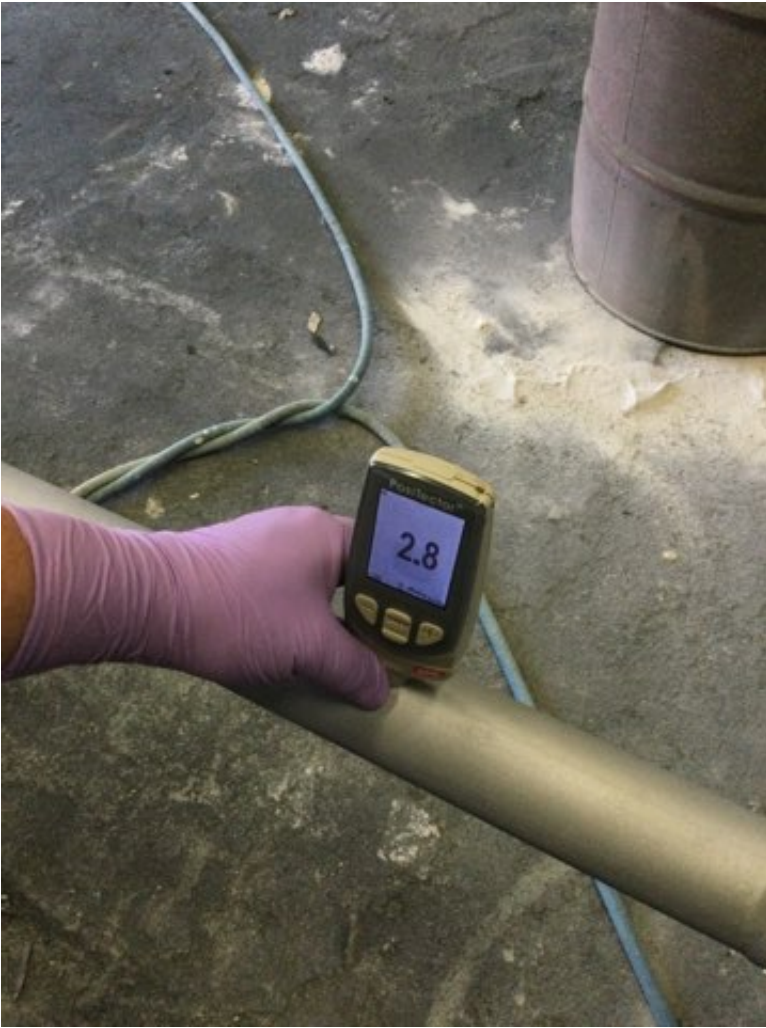
Photo Description: Grit blasted Surface profile measurement
