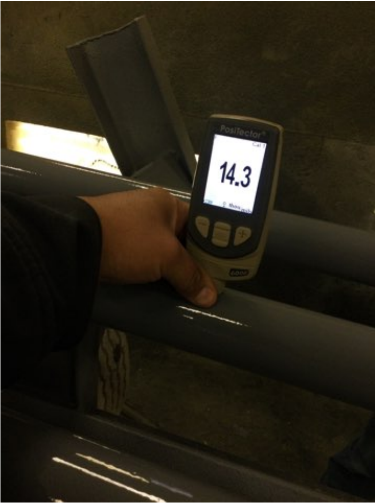
Photo Description: Polyurethane dry film thickness measurement
