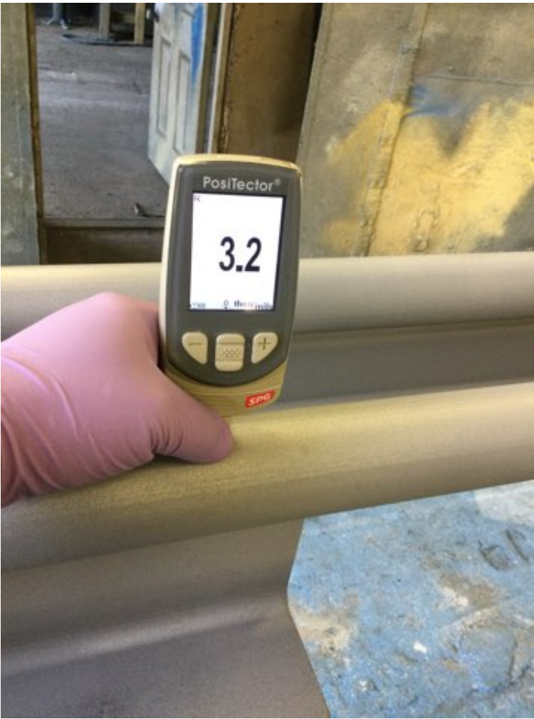
Photo Description: Grit blasted Surface profile measurement
