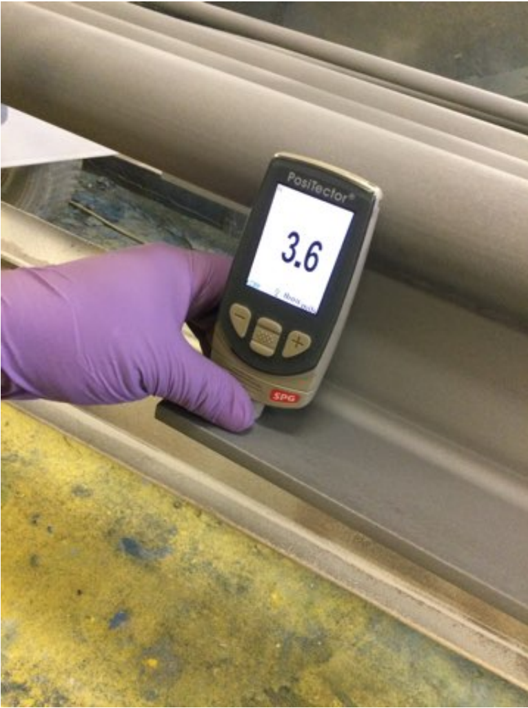
Photo Description: Grit blasted Surface profile measurement
