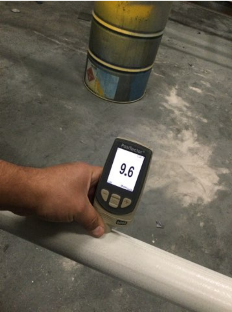
Photo Description: Epoxy dry film thickness measurement
