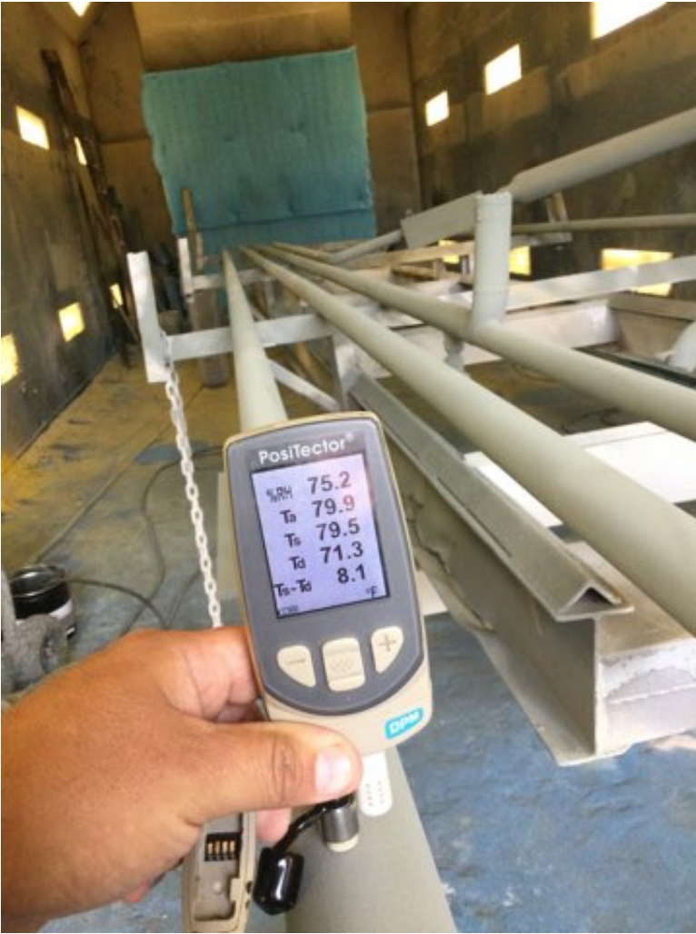
Photo Description: Immediately before Epoxy coating
