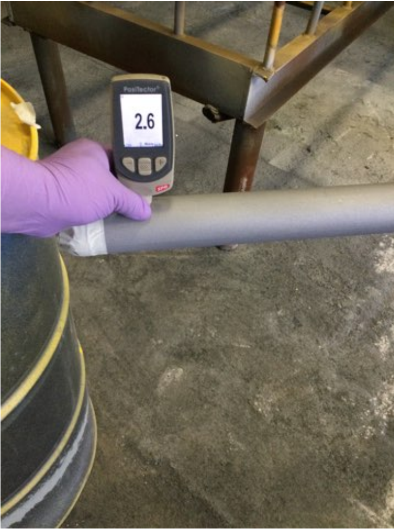
Photo Description: Grit blasted Surface profile measurement
