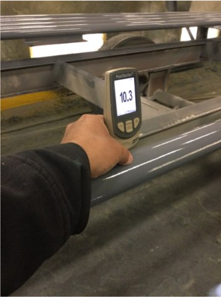
Photo Description: Polyurethane dry film thickness measurement
