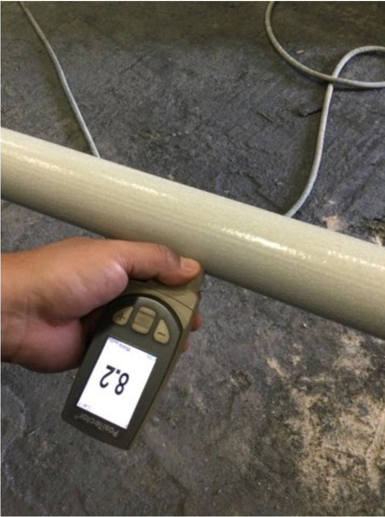
Photo Description: Epoxy dry film thickness measurement
