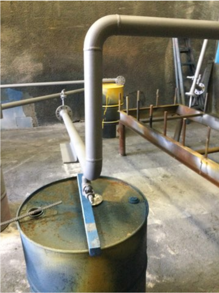
Photo Description: Grit blasted
