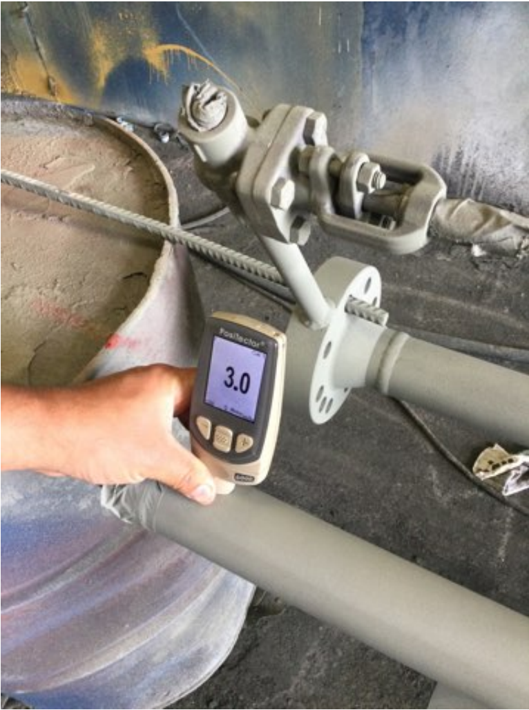
Photo Description: Zinc coating dry film measurement
