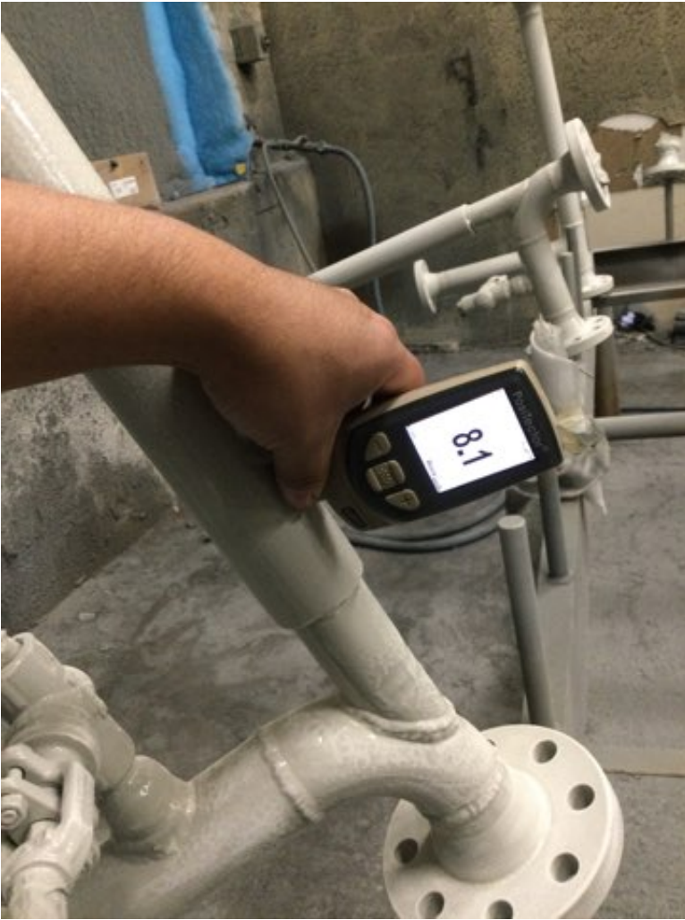
Photo Description: Epoxy dry film thickness measurement
