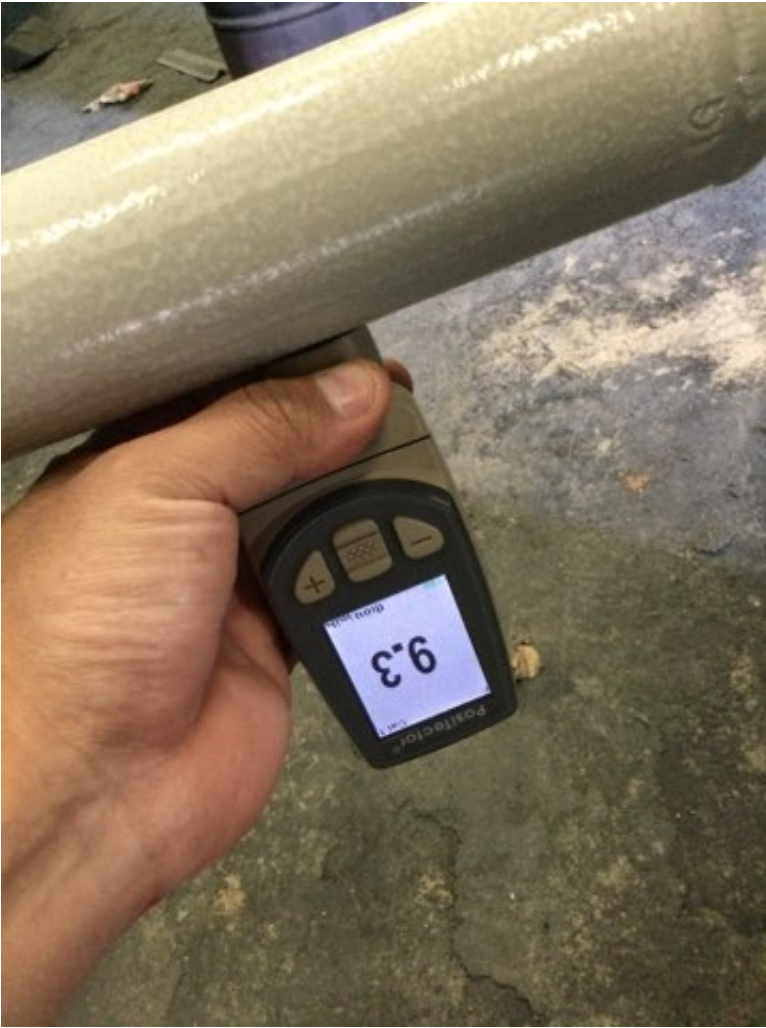
Photo Description: Epoxy dry film thickness measurement
