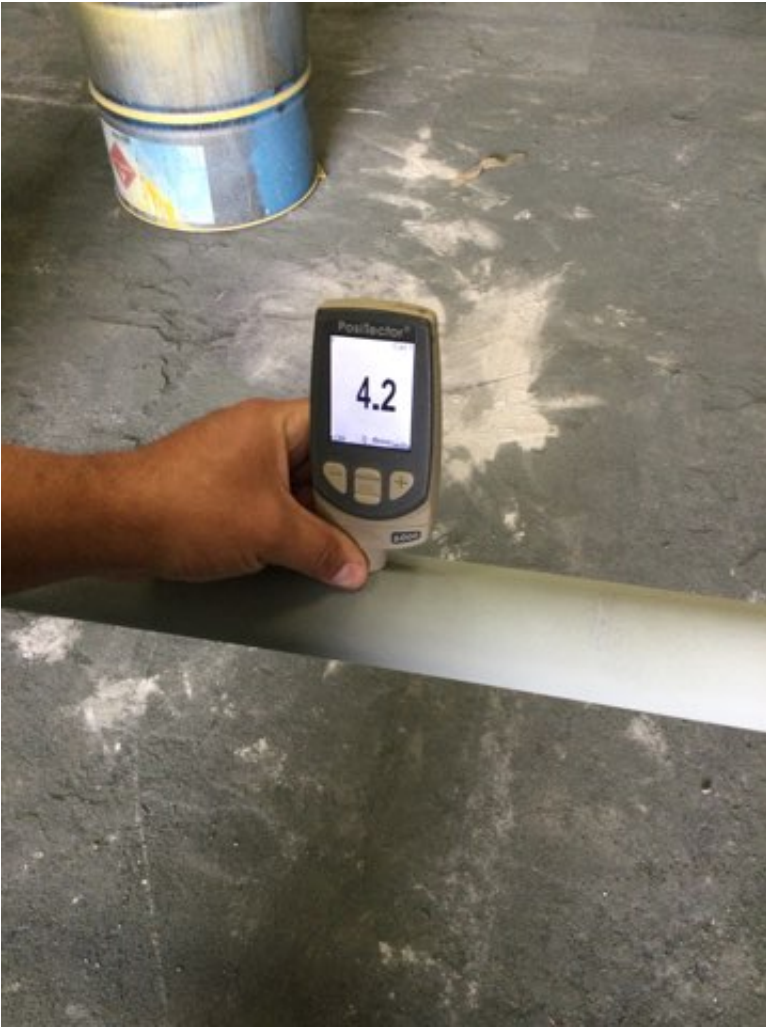
Photo Description: Zinc coating dry film measurement
