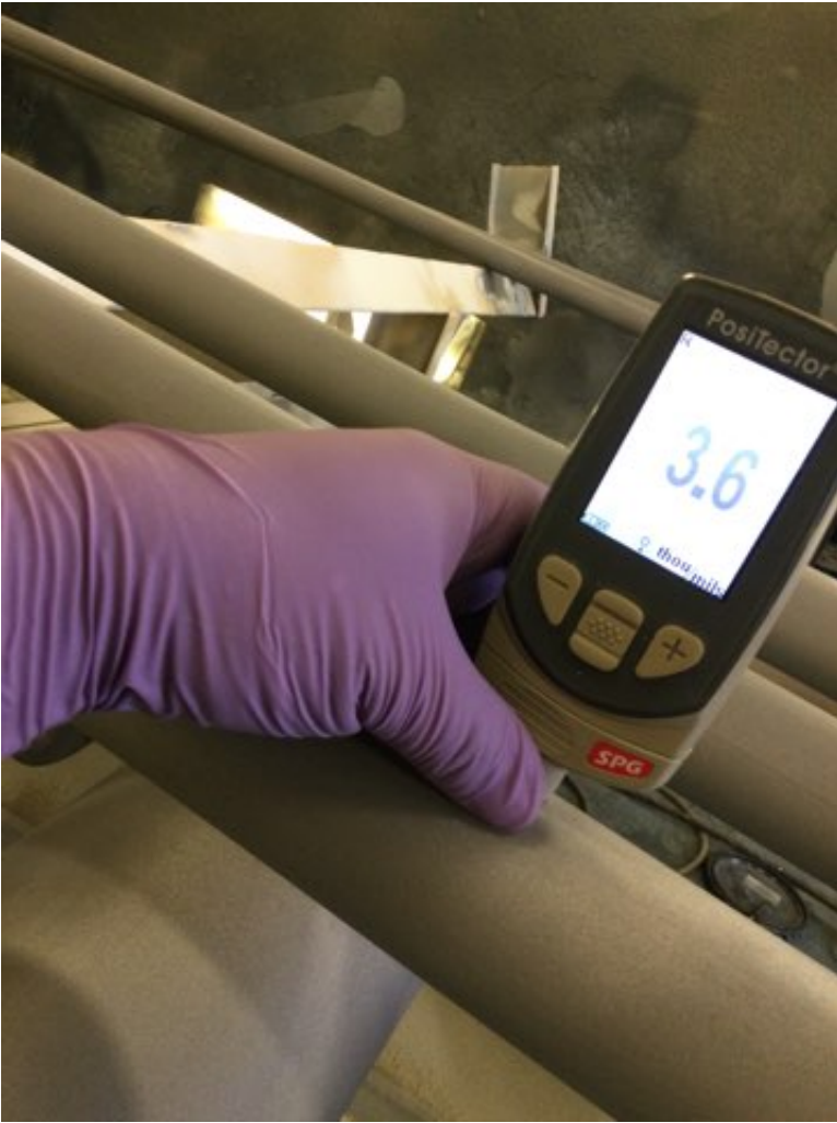
Photo Description: Grit blasted Surface profile measurement
