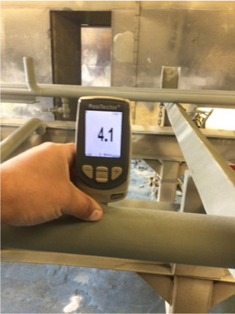
Photo Description: Zinc coating dry film measurement
