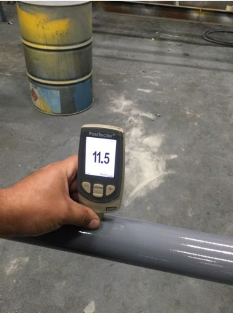
Photo Description: Polyurethane dry film thickness measurement
