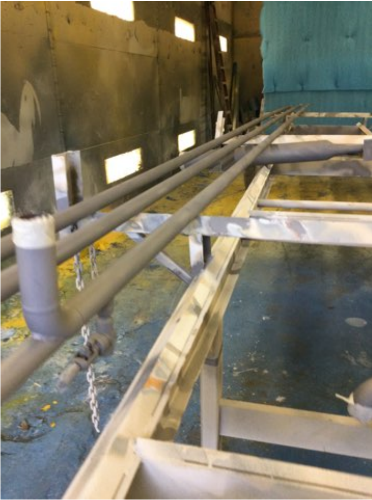
Photo Description: Grit blasted
