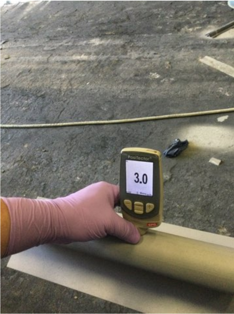
Photo Description: Grit blasted Surface profile measurement
