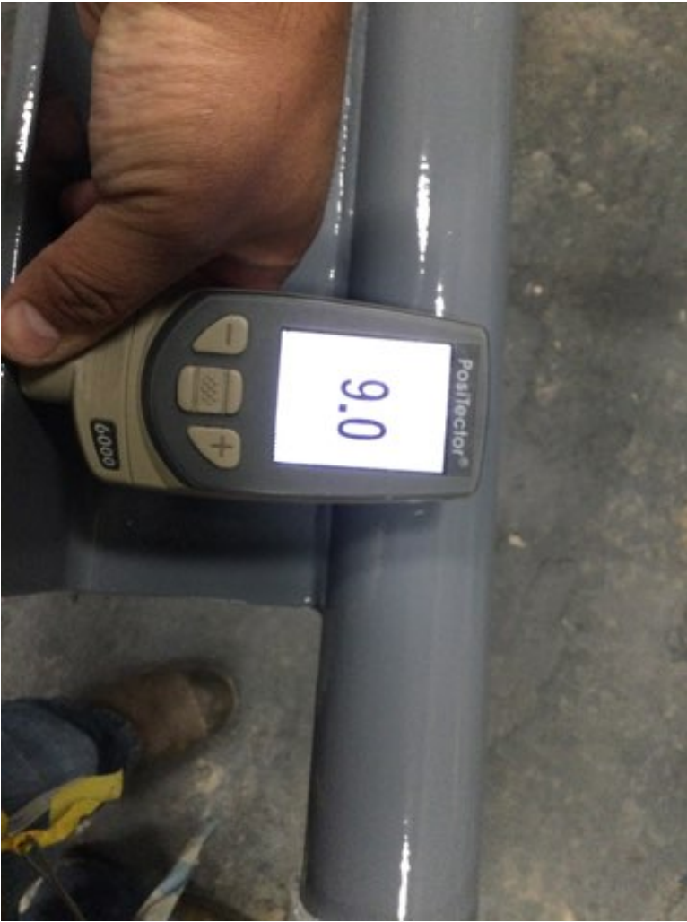
Photo Description: Polyurethane dry film thickness measurement
