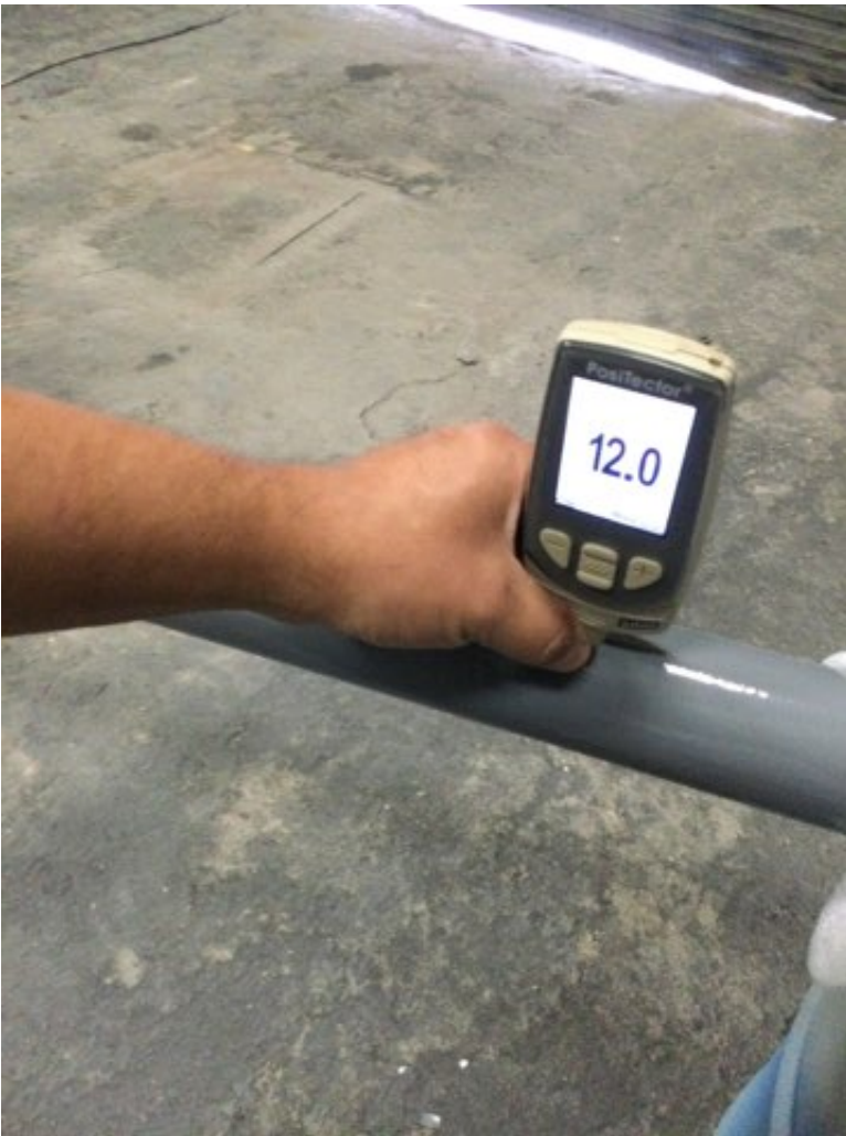
Photo Description: Polyurethane dry film thickness measurement
