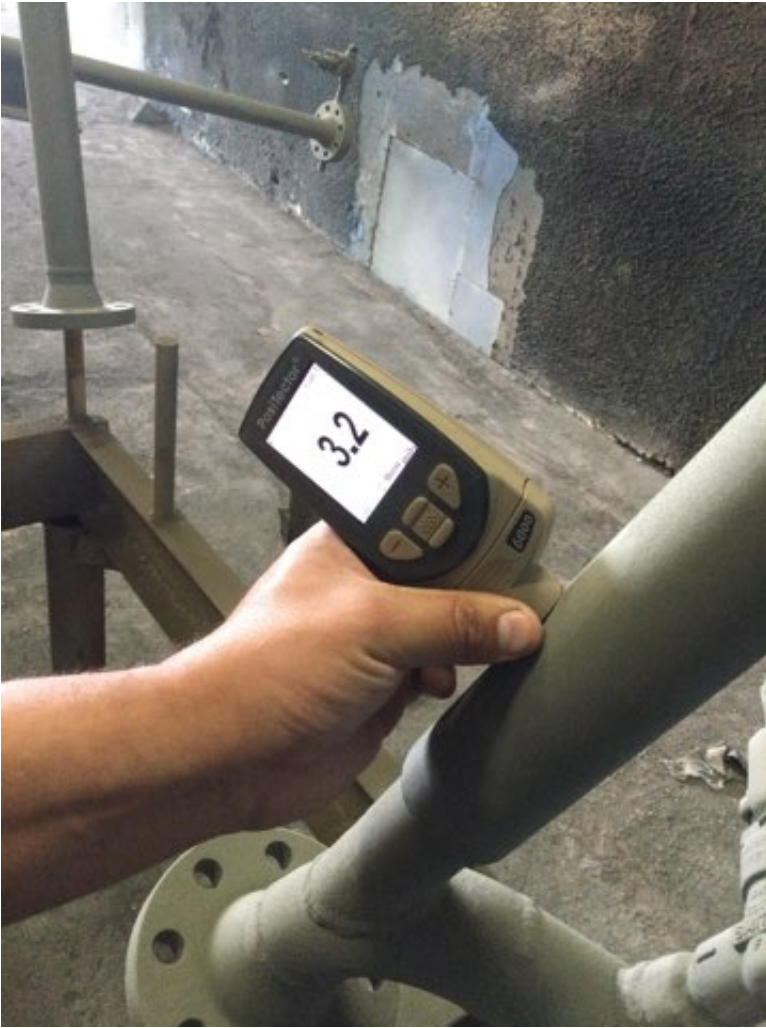
Photo Description: Zinc coating dry film measurement
