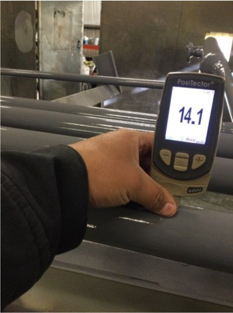
Photo Description: Polyurethane dry film thickness measurement
