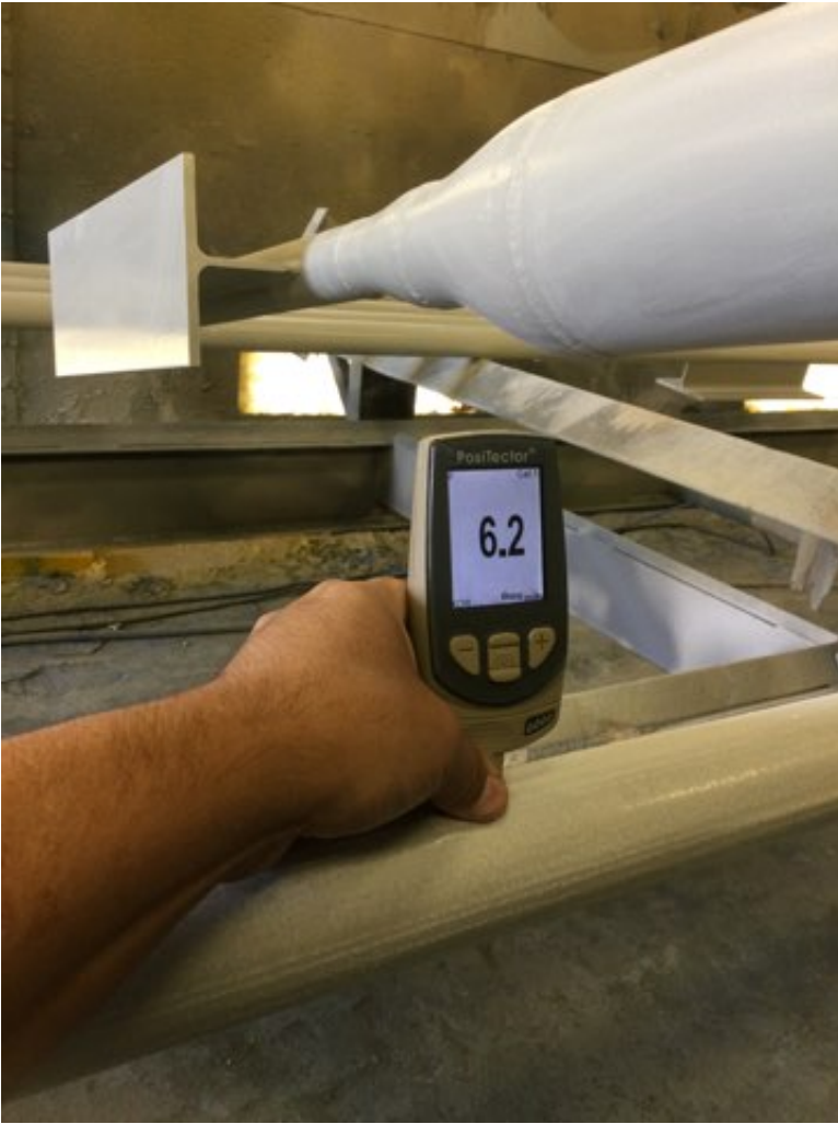
Photo Description: Epoxy dry film thickness measurement
