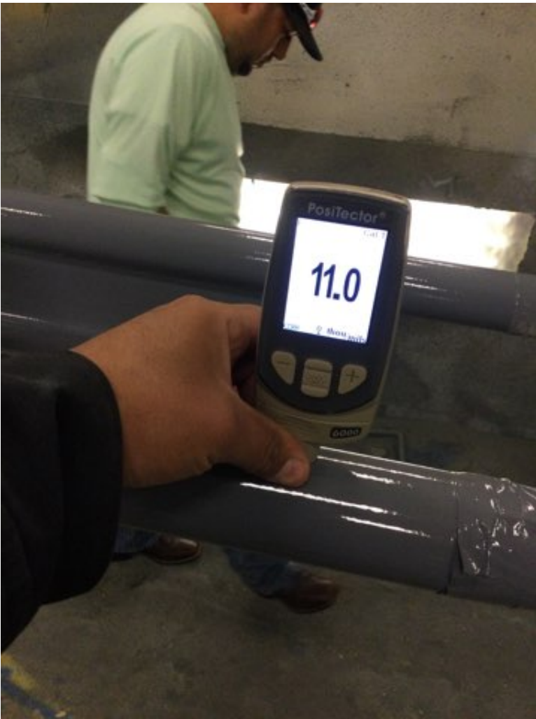
Photo Description: Polyurethane dry film thickness measurement
