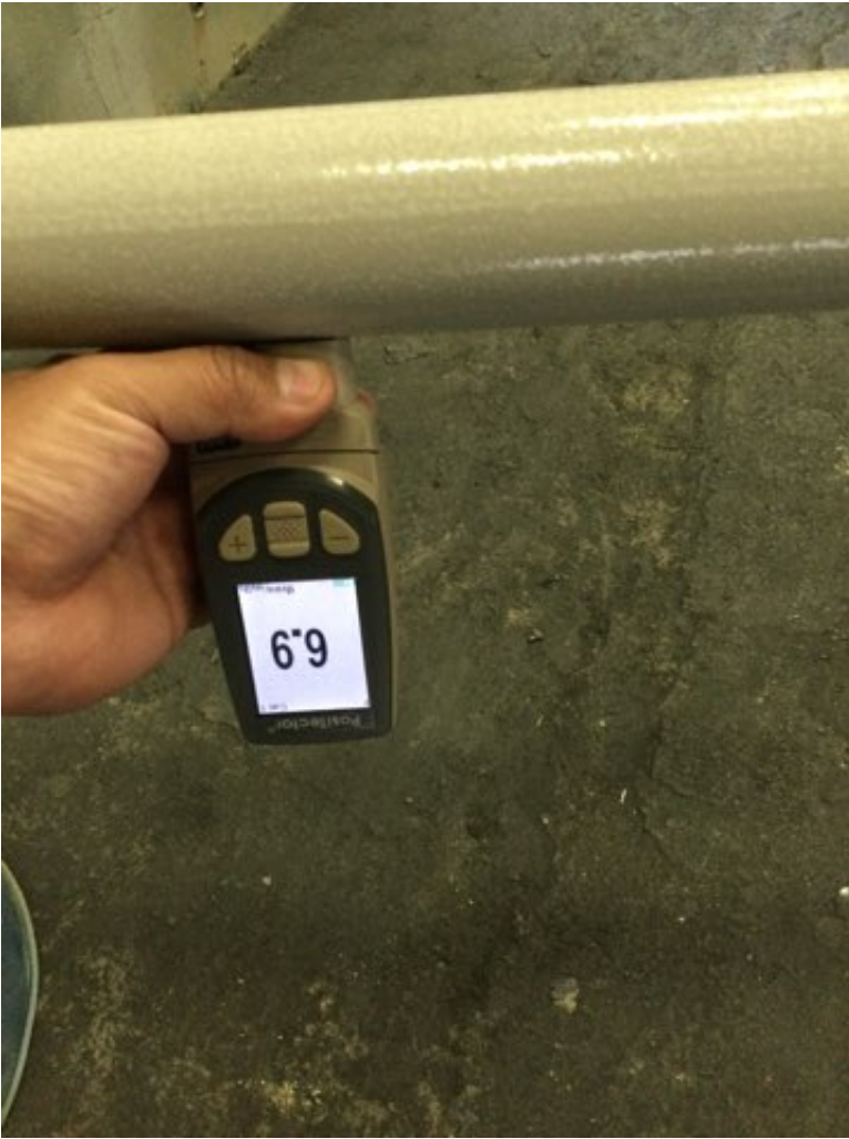
Photo Description: Epoxy dry film thickness measurement
