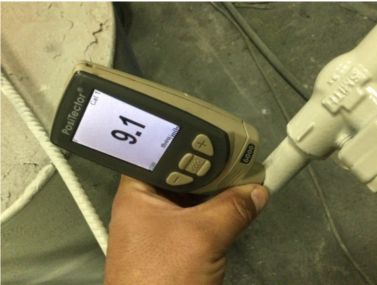
Photo Description: Epoxy dry film thickness measurement
