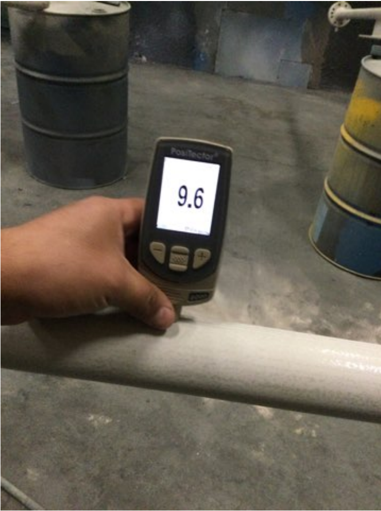
Photo Description: Epoxy dry film thickness measurement
