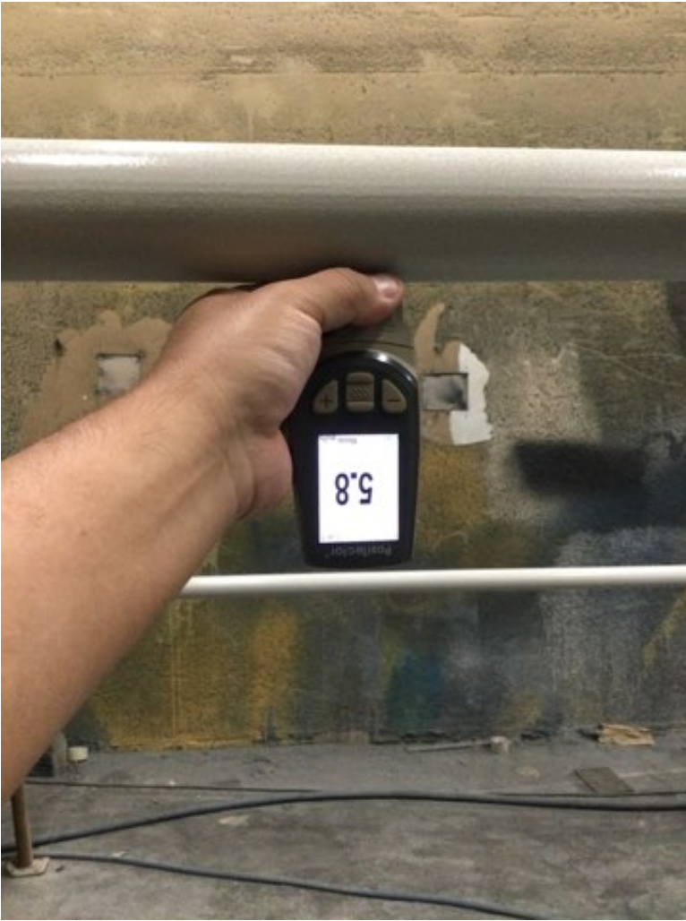
Photo Description: Epoxy dry film thickness measurement
