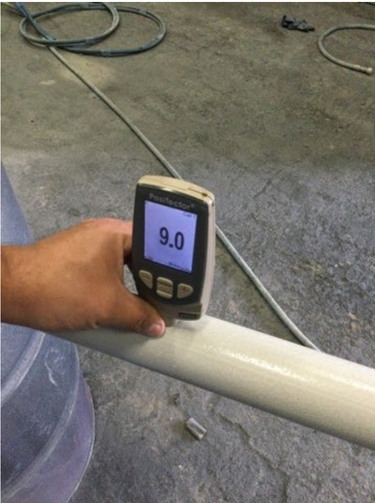
Photo Description: Epoxy dry film thickness measurement
