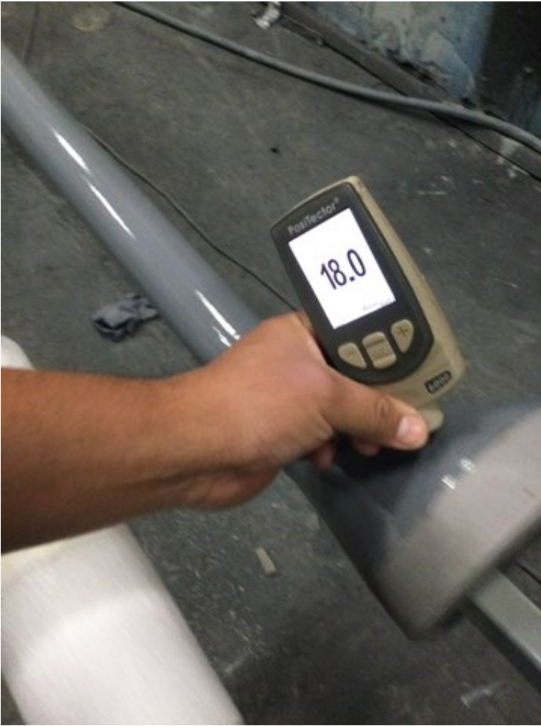
Photo Description: Polyurethane dry film thickness measurement
