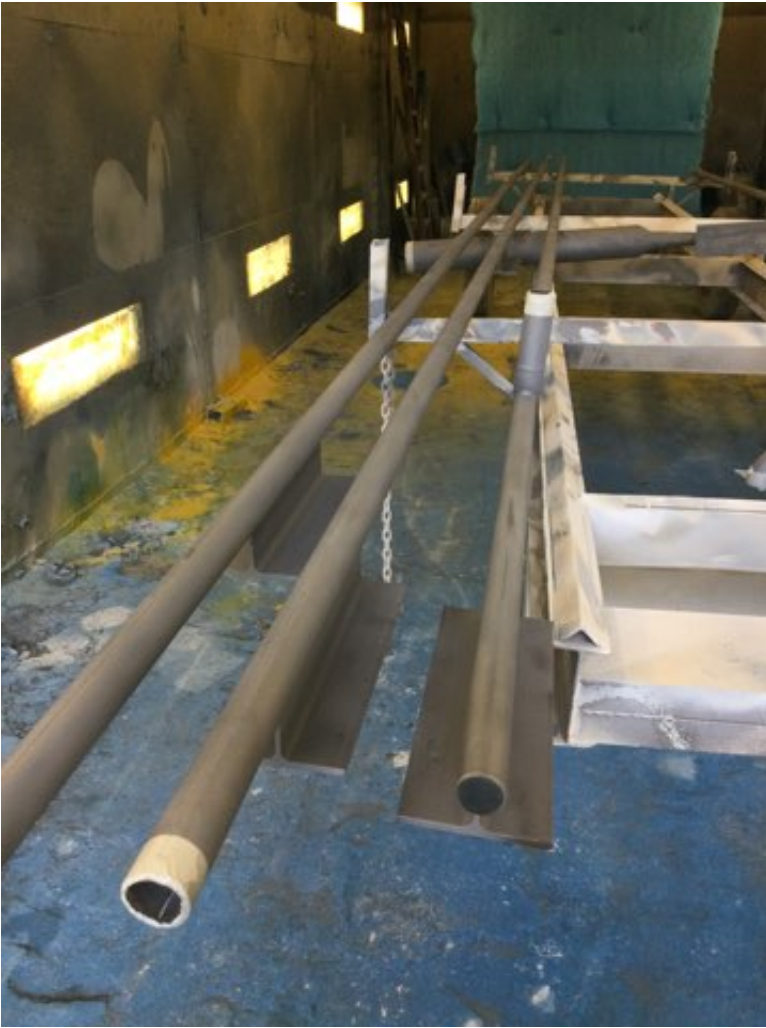
Photo Description: Grit blasted
