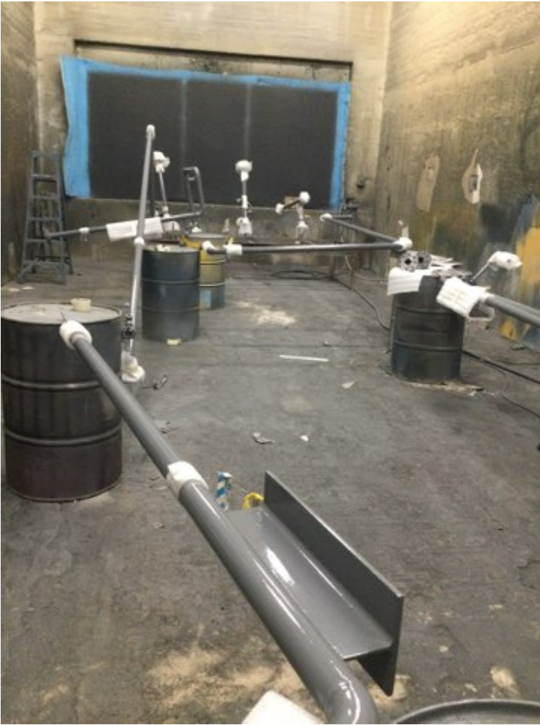
Photo Description: Grey top coat coated
