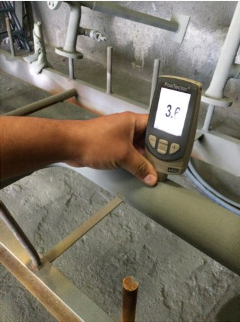
Photo Description: Zinc coating dry film measurement
