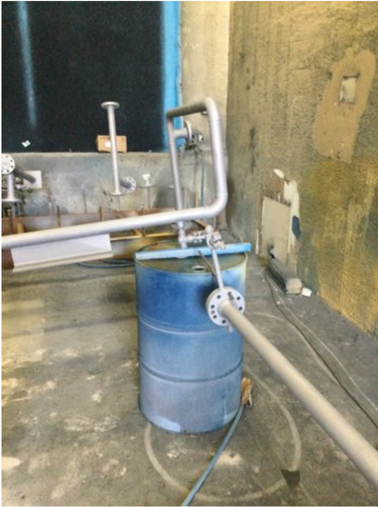
Photo Description: Grit blasted
