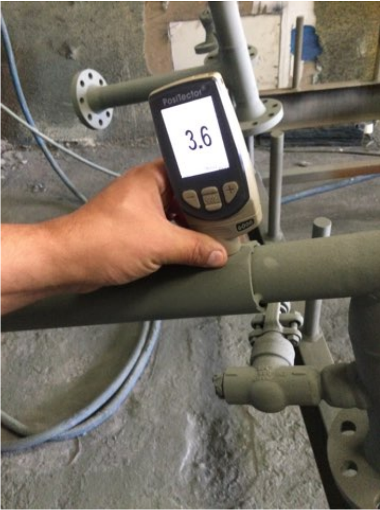
Photo Description: Zinc coating dry film measurement
