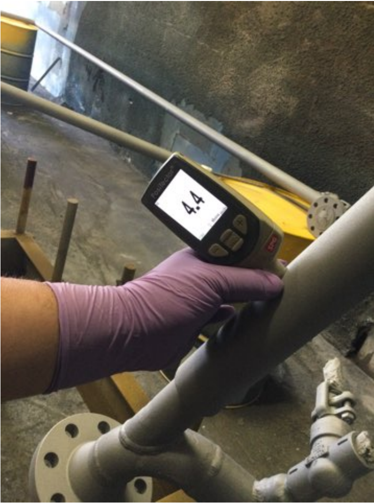
Photo Description: Grit blasted Surface profile measurement
