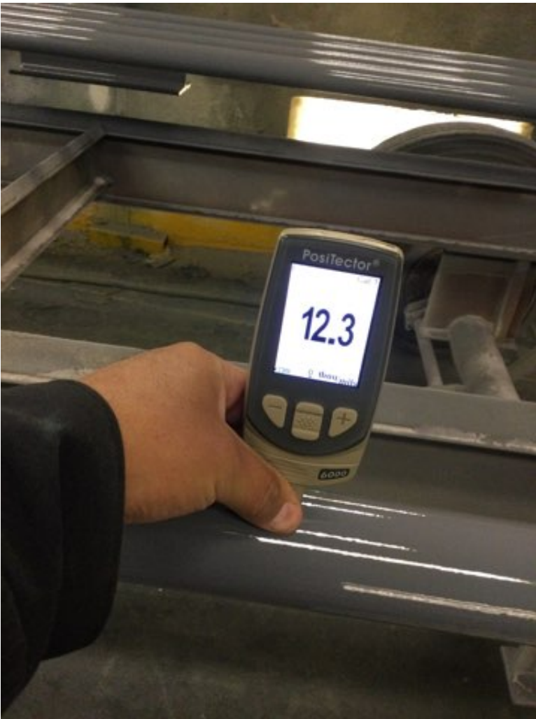
Photo Description: Polyurethane dry film thickness measurement
