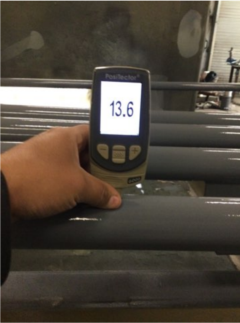
Photo Description: Polyurethane dry film thickness measurement
