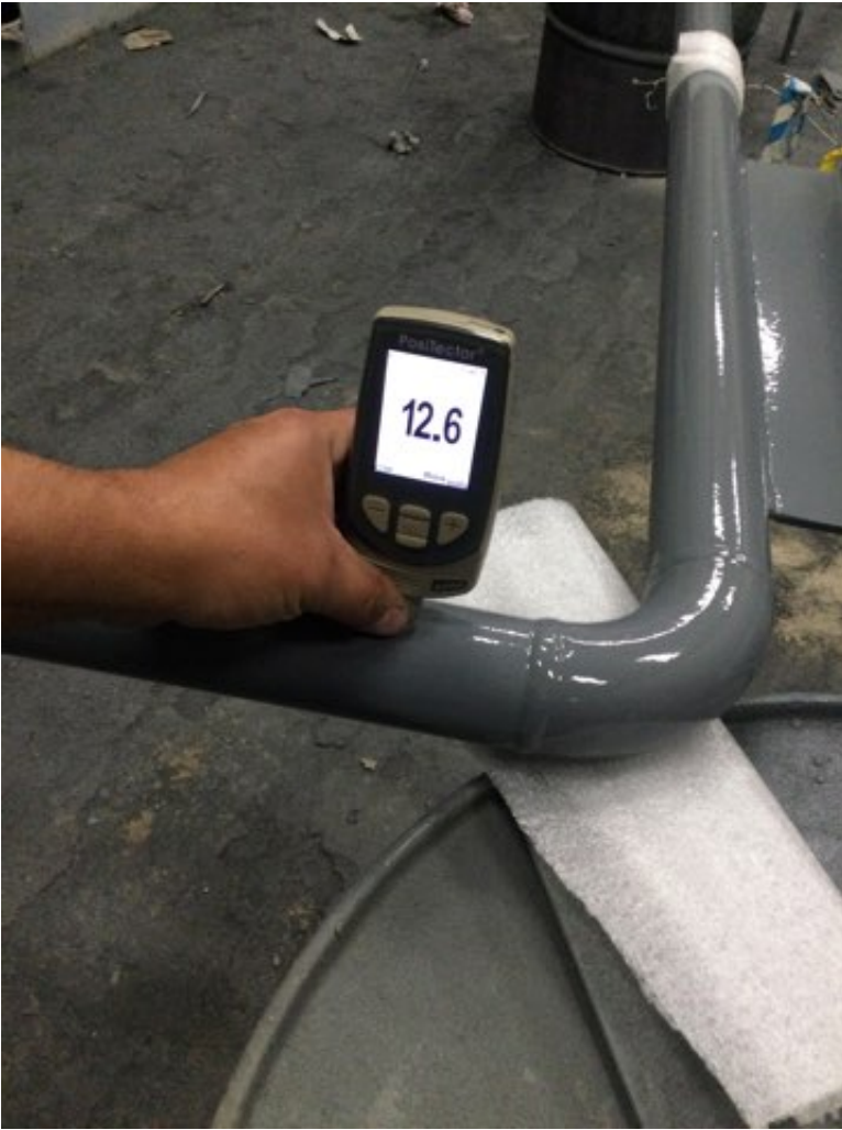
Photo Description: Polyurethane dry film thickness measurement
