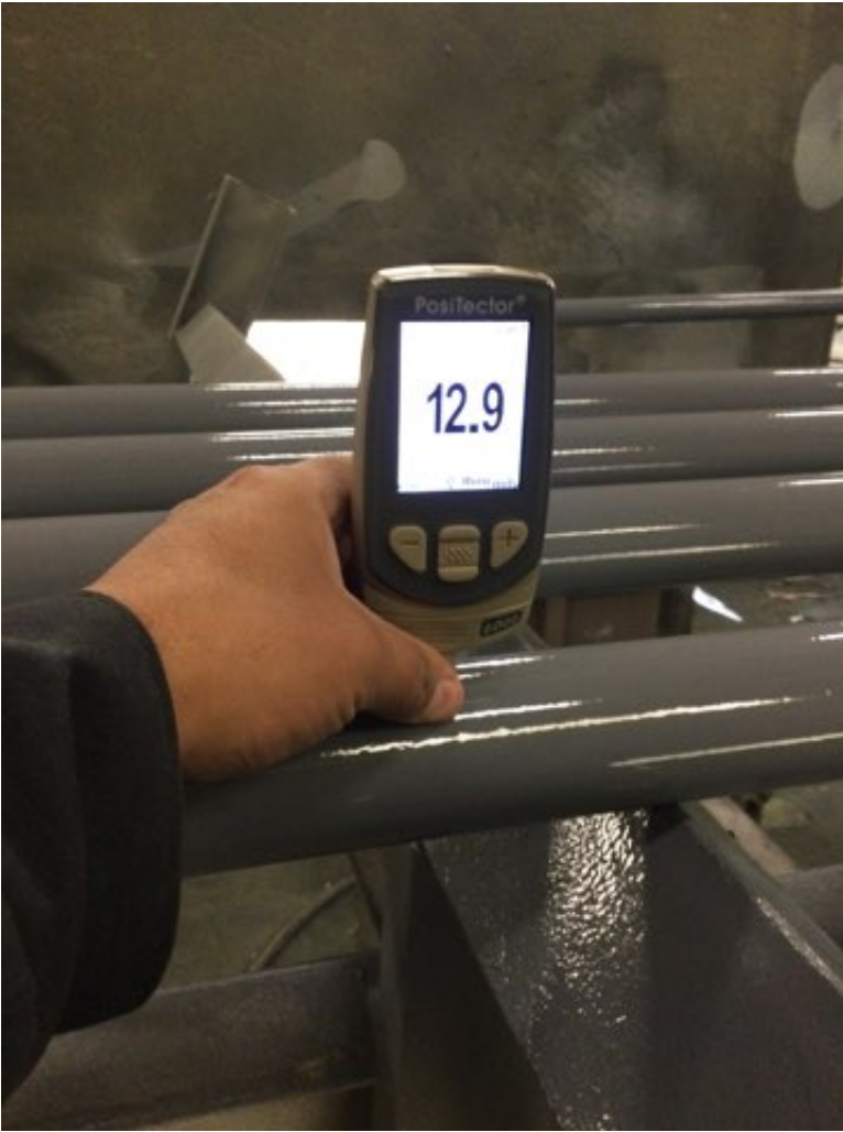
Photo Description: Polyurethane dry film thickness measurement
