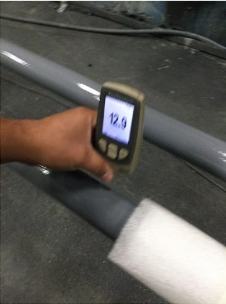
Photo Description: Polyurethane dry film thickness measurement
