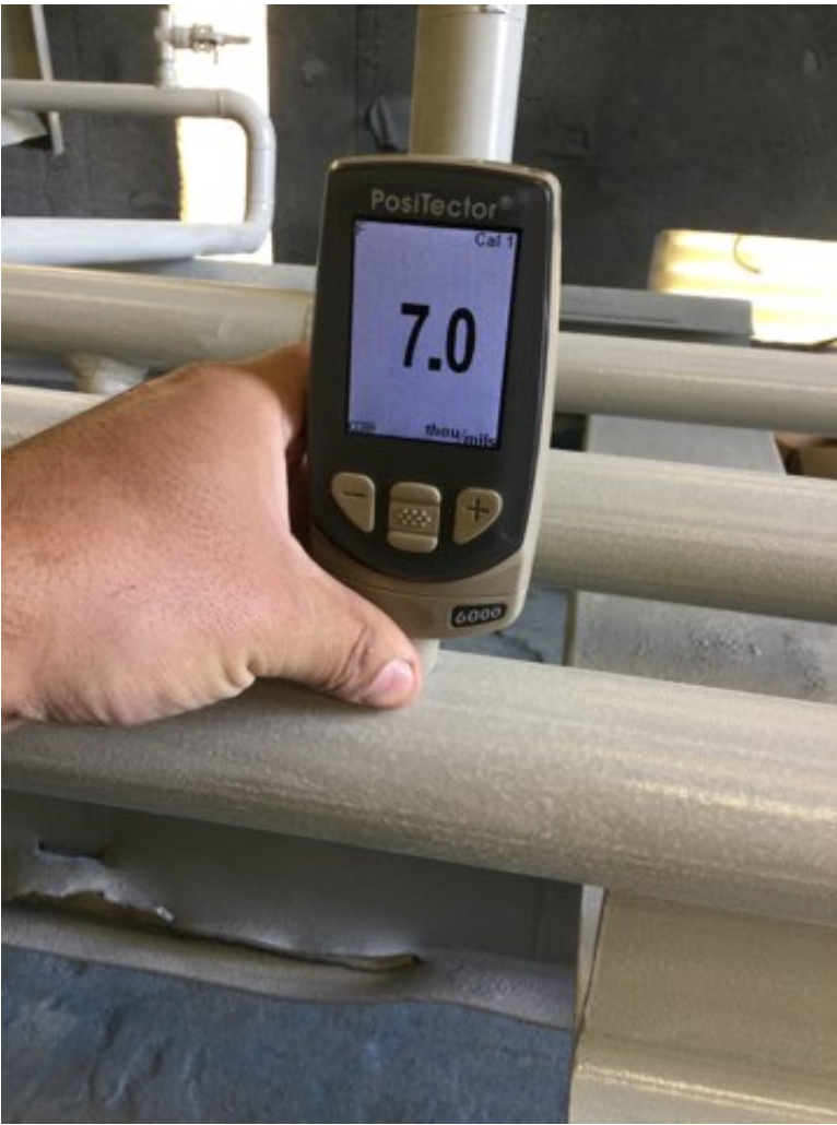
Photo Description: Epoxy dry film thickness measurement
