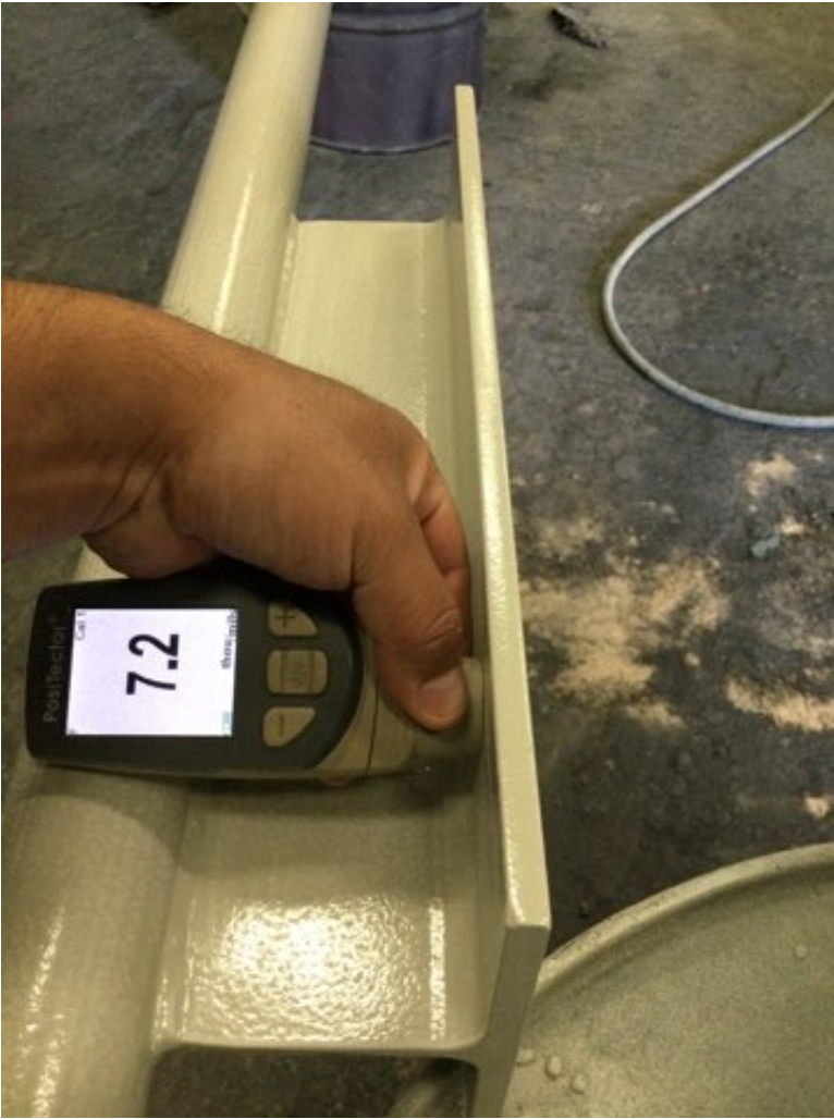
Photo Description: Epoxy dry film thickness measurement
