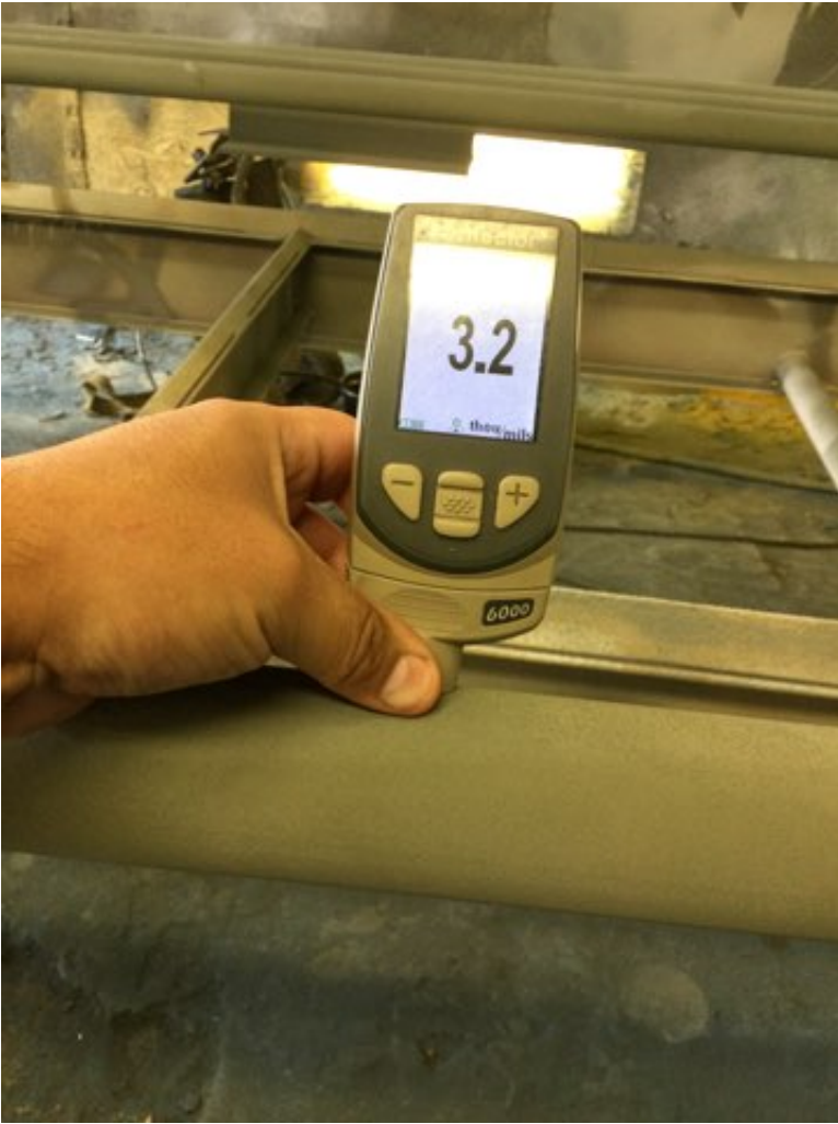
Photo Description: Zinc coating dry film measurement
