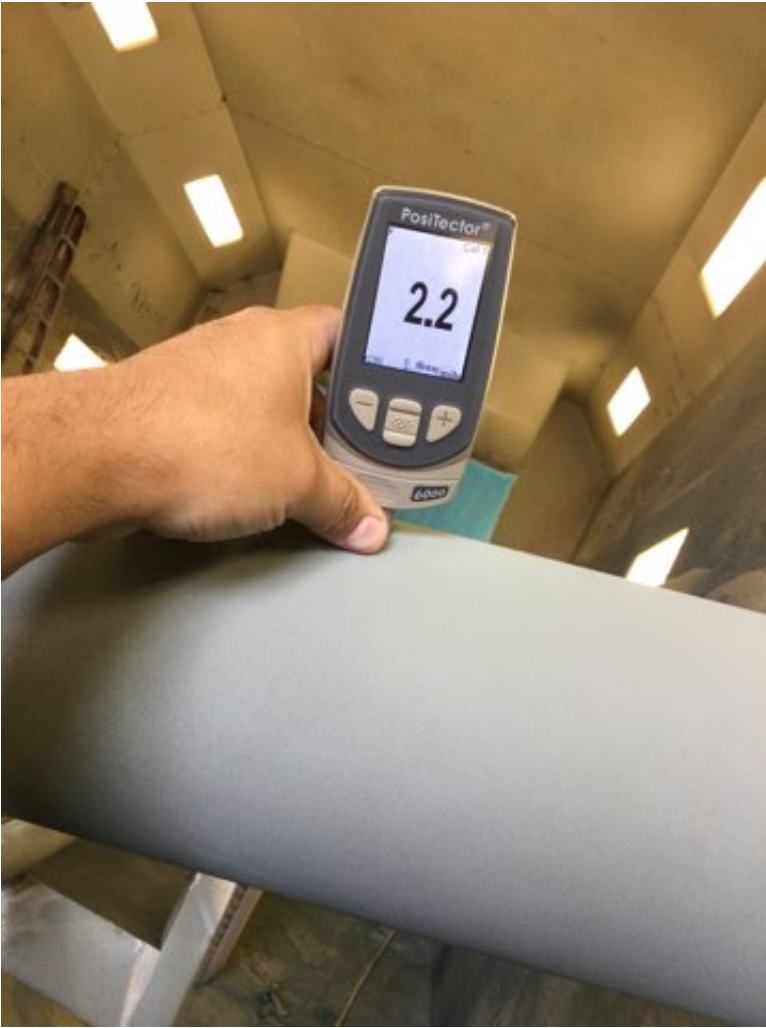
Photo Description: Zinc coating dry film measurement
