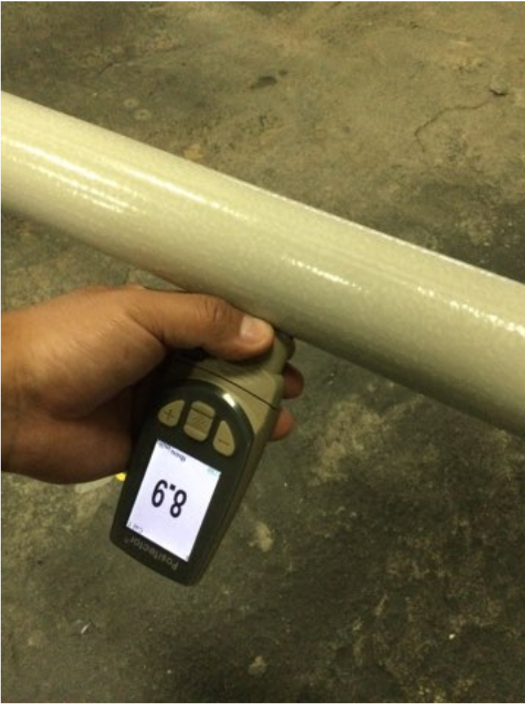
Photo Description: Epoxy dry film thickness measurement
