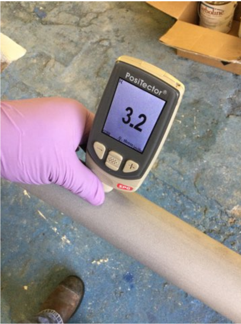
Photo Description: Grit blasted Surface profile measurement
