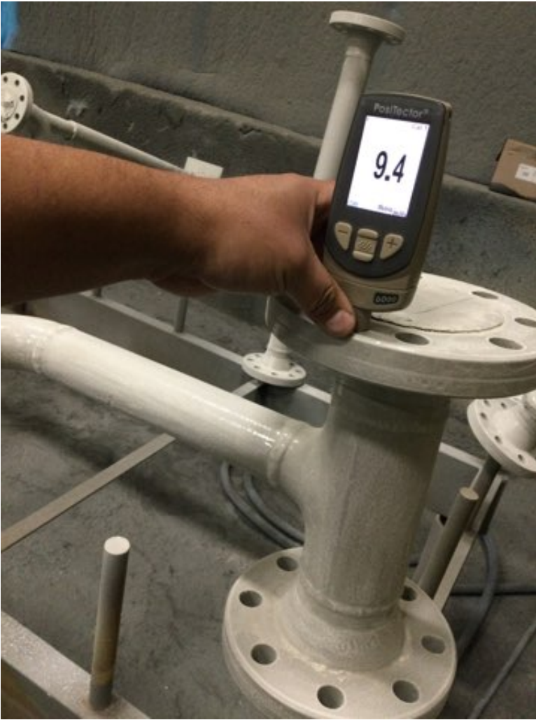
Photo Description: Epoxy dry film thickness measurement
