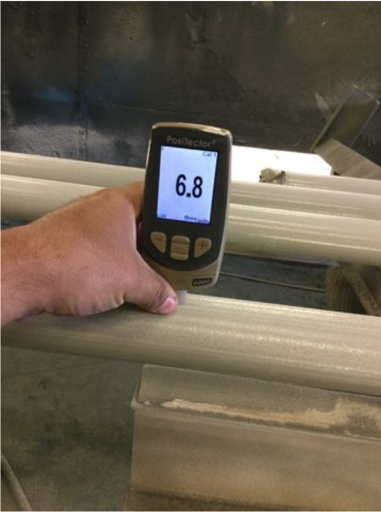
Photo Description: Epoxy dry film thickness measurement
