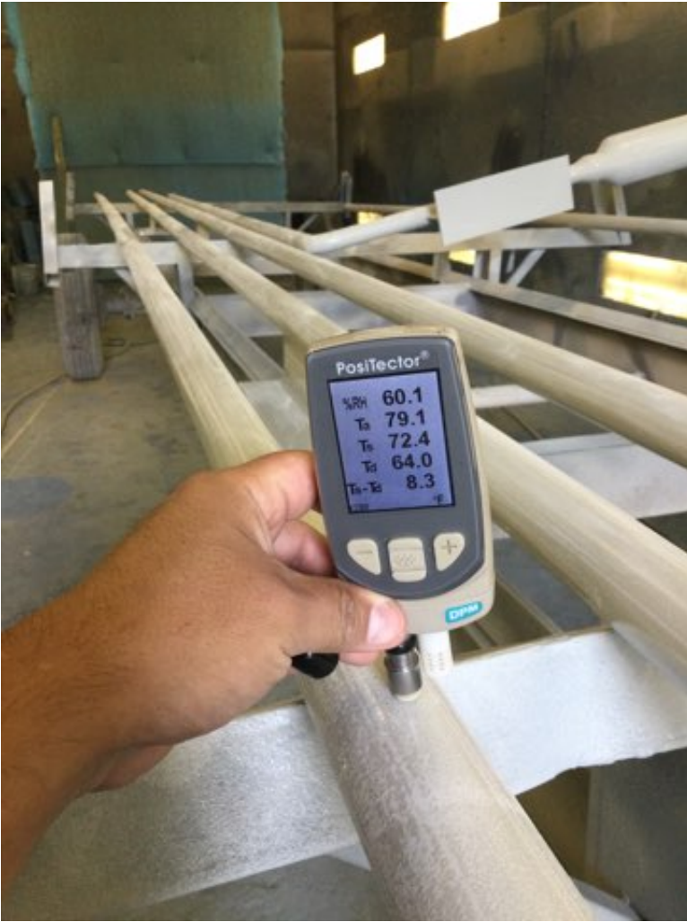
Photo Description: Immediately before polyurethane top coating
