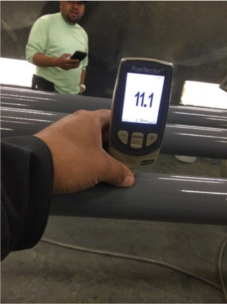
Photo Description: Polyurethane dry film thickness measurement
