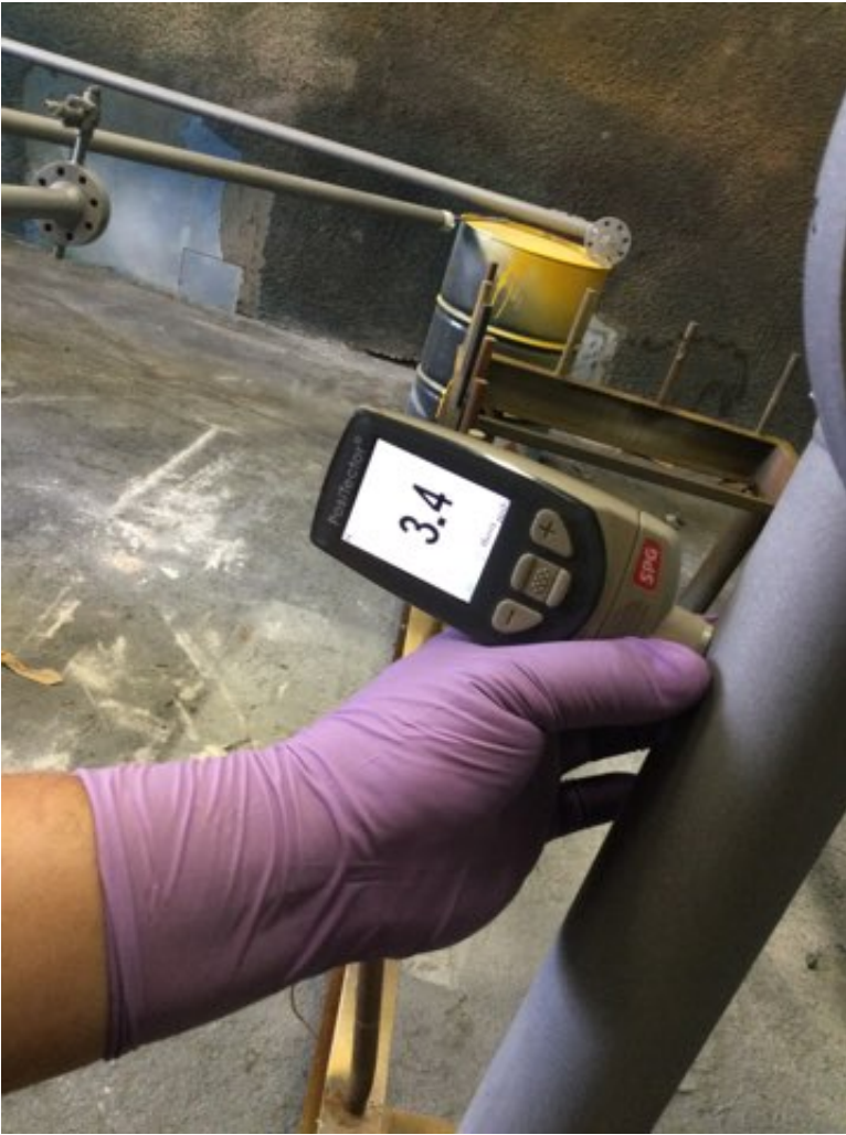
Photo Description: Grit blasted Surface profile measurement
